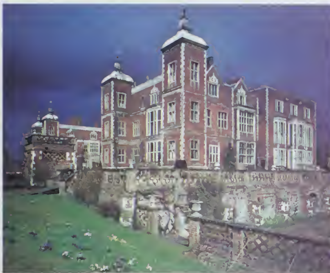
Hatfield House, Hertfordshire
